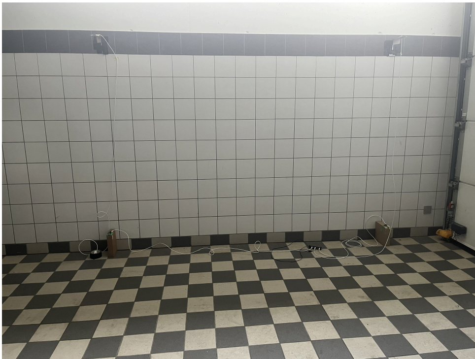
Figure 52: Four of the eight UWB anchors mounted on the wall of the test room.
