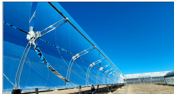
Figure 1: Eurotrough collector at the Plataforma Solar de Almería Own presentation
