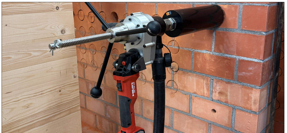
Drilling test on masonry Own presentation
